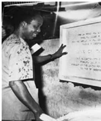
On the left hand side, the first President of the United Republic of Tanzania, Mwalimu Julius K. Nyerere laying the foundation stone of the Bank of Tanzania headquarters in Dar es Salaam on 9th December 1966.
