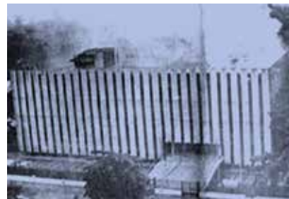
The Bank's headquarter building on fire on 17 th May 1984
