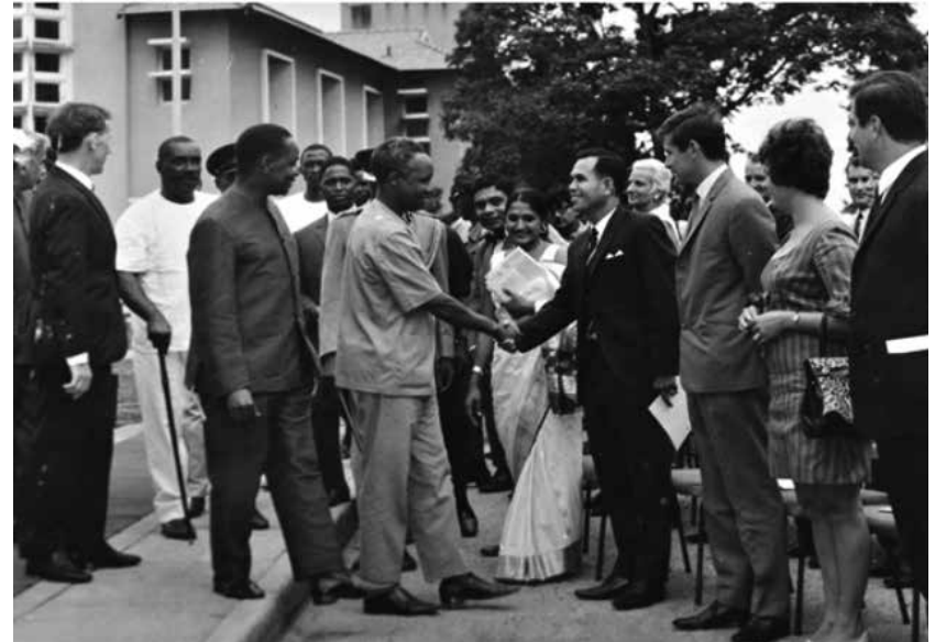
Mwalimu Nyerere shaking hands with the contractor of the Bank's first headquarters building on 9th December 1966. Others in the photo include the first President of the Revolutionary Government of Zanzibar, Mr. Abeid Amani Karume (holding a walking stick) and the first Bank of Tanzania Governor, Mr. Edwin Mtei (on the right hand side of Mwalimu Nyerere).
