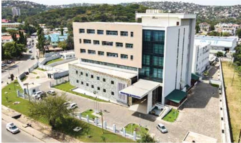
The Bank of Tanzania's Mwanza Branch building
