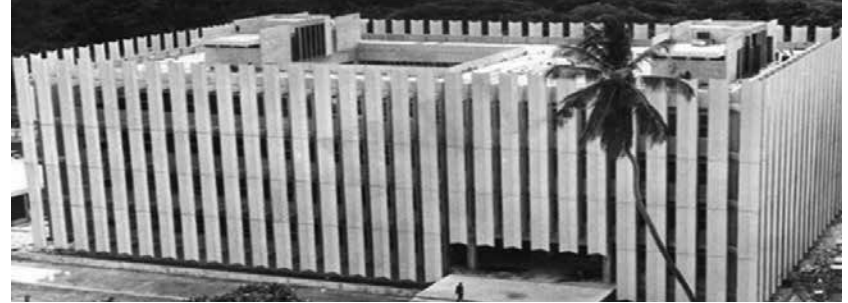
The Bank's headquarter building (1969)
